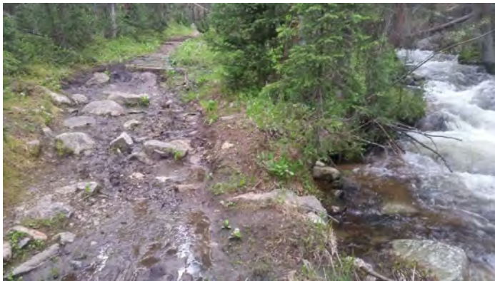
Before CTF Volunteers - wet & eroded
